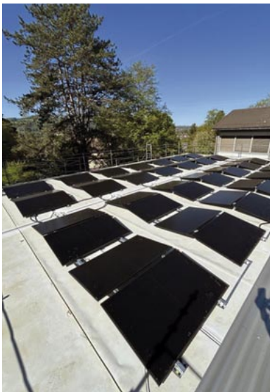
Mobile Photovoltaik-Anlage. Bilder: zVg
